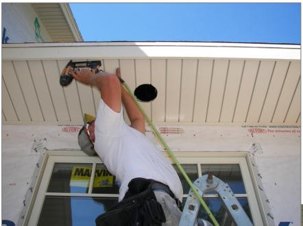
3. Install panel(s) and reinstall grille with vanes directing air 'away from' the building:
