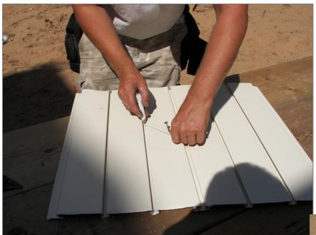
2. Locate the correct position in the soffit panel(s) and cut the hole:
